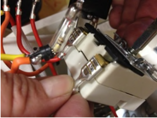
Figure 10. Unplug two connections from thermostat base found inside sealer head
