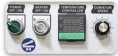
Tunnel Control Panel
