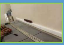
15. For best results, manually attach screw and double check if bar is level.
