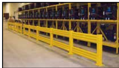
Guarding Battery Racks
