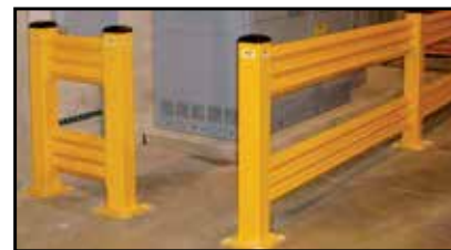
Guarding Electrical Panels
