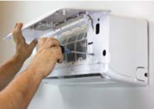
Back out electrical panel screws
