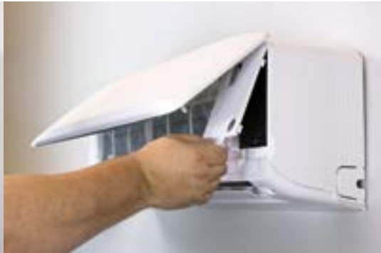
Remove electrical access panels (2)
