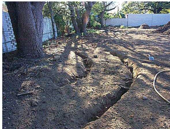
Trenches are being located around this existing tree to accommodate an electrical conduit.
