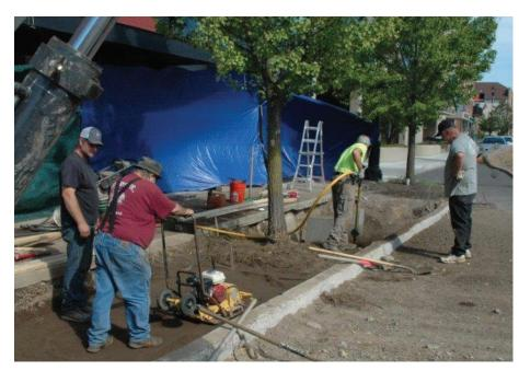
Installation of a new paving system for ginko street trees. At the right of the photo, an arborist excavates highly compacted sandy loam soil that had supported brick pavement for over 20 years. At left, the contractor finishes installation of an engineered sand based structural soil, which is to bear the load of new pavement.
