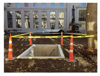
To install this area-way at M.I.T. required diligent tree protection, and intensive excavation using an AirSpade and root pruning by a trained arborist. (Image courtesy of SSA.)
