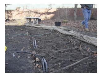
At the Radcliffe Institute, the foundation for a new path was excavated using an AirSpade. Irrigation lines were snaked through the exposed roots, and minimal root pruning was completed before installing a gravel root barrier and the top course of stone dust pavement. (Image courtesy of SSA.)
