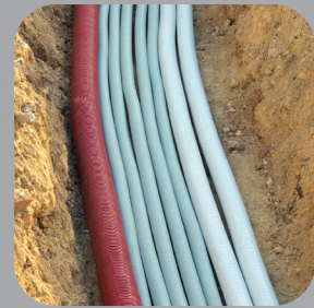
Electric Power Lines
