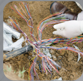
Telecommunication Lines and Fiber Optics
