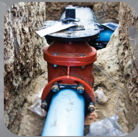
Water and Sewer Lines
