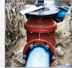
Water & Sewer Lines
