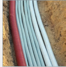
Electric Power Lines
