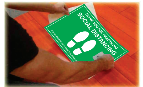
STEP 6: Squeegee down part of the decal in a vertical motion.
