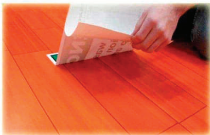
STEP 7: Remove the rest of backing paper.
