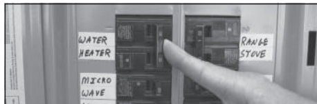
Figure 22 - Circuit Breaker
